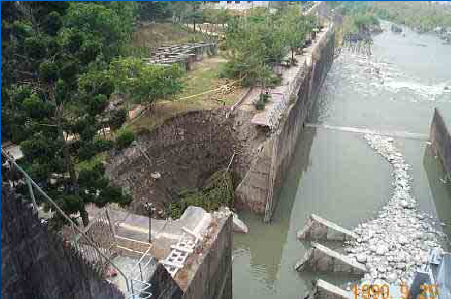
Retaining wall failure at the Shin-Kang Dam
