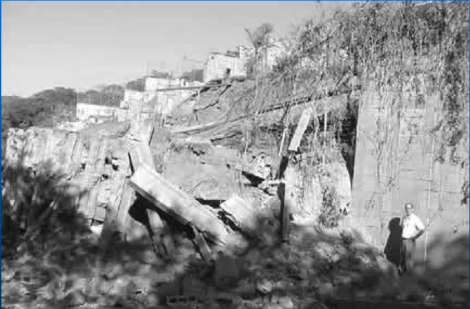
retaining wall failure during earthquake
